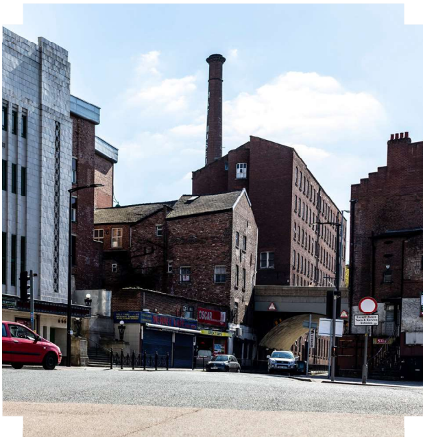
The town centre is peppered with red-brick mills, warehouses and infrastructure serving as a reminder of our rich industrial heritage | Former Wellington Mill, Wellington Road South (A6)
