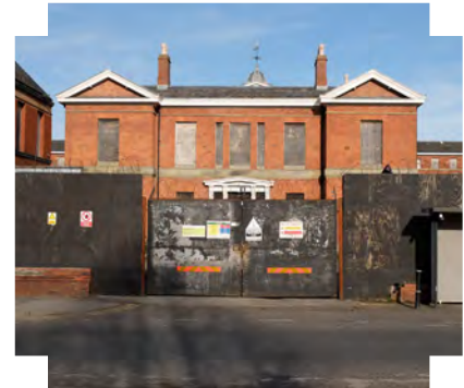
St Thomas' Hospital buildings
