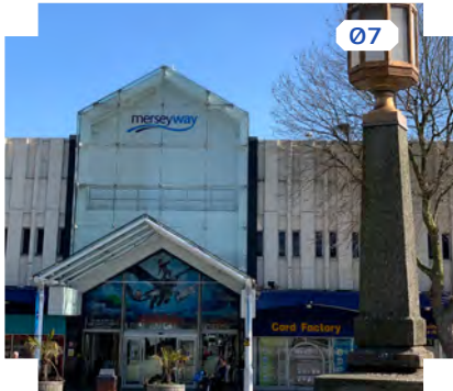
Merseyway Shopping Centre
