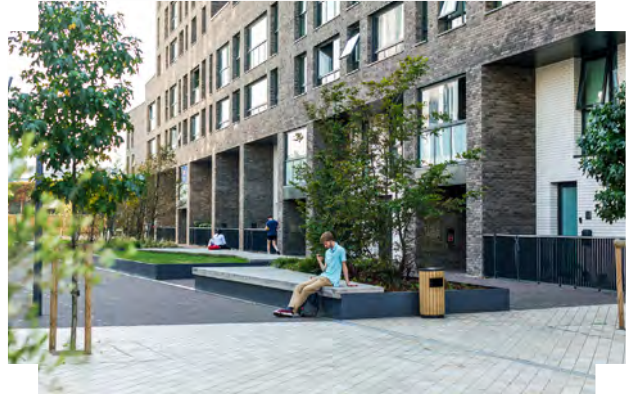
Raised crossing points, tree planting and street furniture create a safer pedestrian environment along the street | Elephant Park, London
