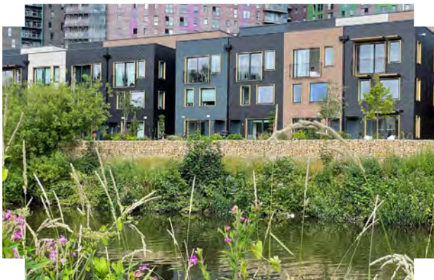
Homes adjacent to the river are raised above the river corridor using a biodiverse sloping buffer Climate Innovation District, Leeds
