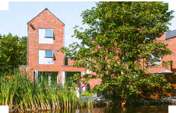
Prominent gables and large windows address the riverfront | The Oaks, Crosby
