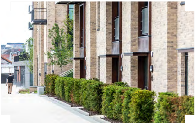
Large windows and front doors address the street, with a low hedgerow boundary ensuring a visual connection between home and street | Middlewood Locks, Salford
