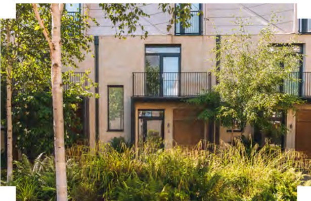
Space for cycle and bin storage integrated into the entrance area of the townhouse, well-overlooked by windows above | Bath Riverside, Bath
