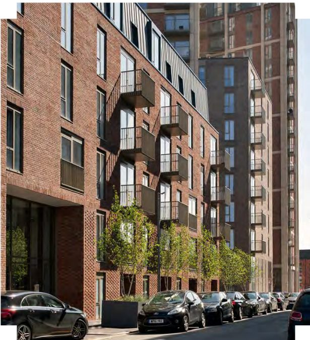
Two-storey townhouses with front doors address the street, with apartments located above
