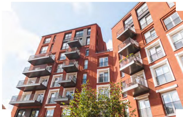
A range of architectural features create depth and interest in the elevation, including balconies, deep reveals, mixed secondary materials and stepped building heights | Keybridge House, London
