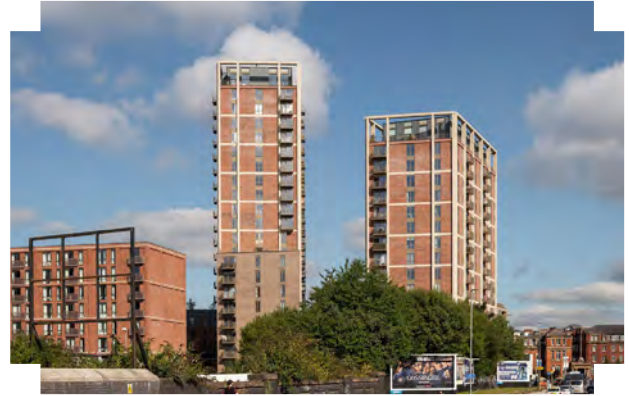
Well-proportioned and stepped buildings define the city gateway | The Crescent, Salford (5Plus Architects)
