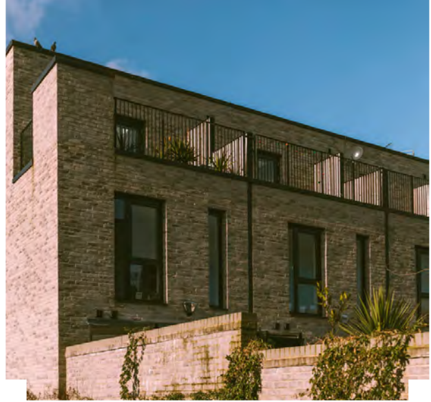
Subtly integrated roof terraces Timekeepers Square, Salford
