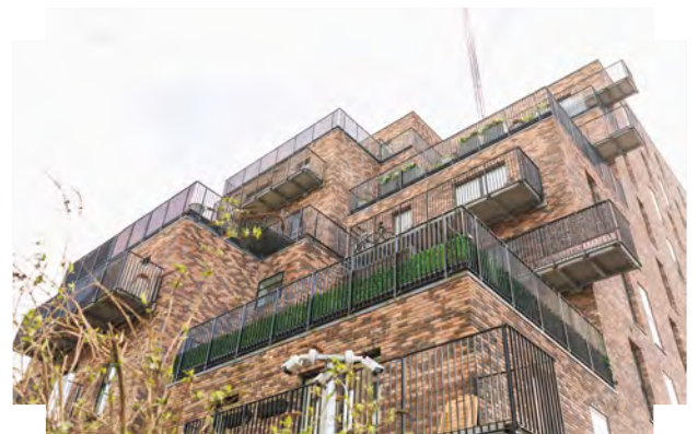
Large roof terraces create opportunities for rainwater harvesting, planting and solar panels New Islington, Manchester
