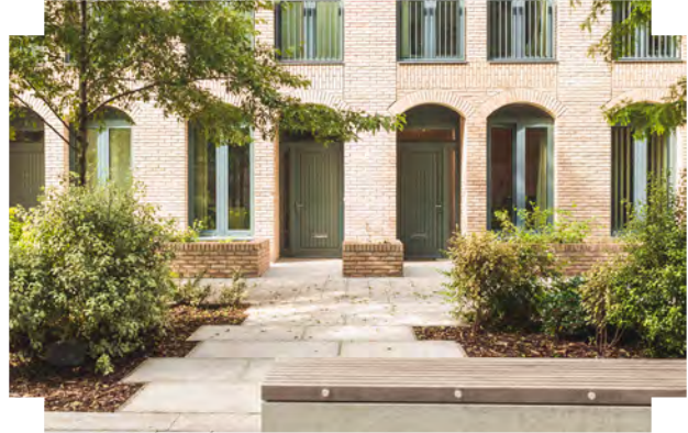
A narrow threshold, low boundary and recessed building entrance protect the privacy of residents and reinforce a fine urban grain | Embassy Gardens, London
