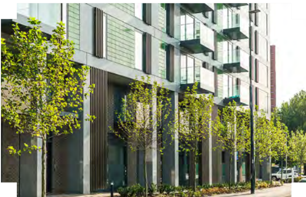
Double-height ground floor, recessed entrances and tree planting creates a threshold and protects residents' privacy | Blackfriars, Salford
