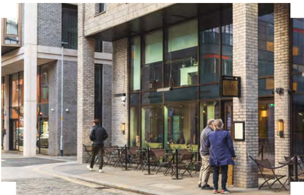
Tall and transparent ground floor, recessed to create covered spill-out space for businesses | Ancoats, Manchester
