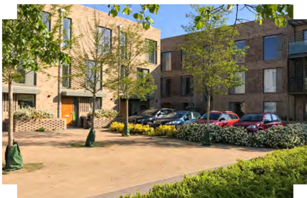
Car parking designed to the edge of communal courtyard maximises the amenity value of the space Great Kneighton, Cambridge
