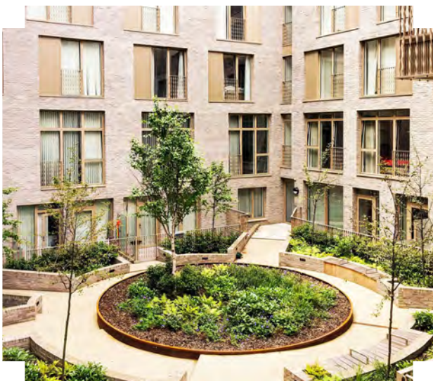
Windows and doors address a green communal courtyard (Photography © Simon Kennedy)
