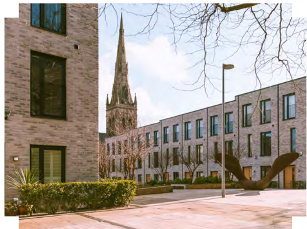
A holistic materials palette creates a positive relationship between homes and the public realm | Timekeepers Square, Salford
