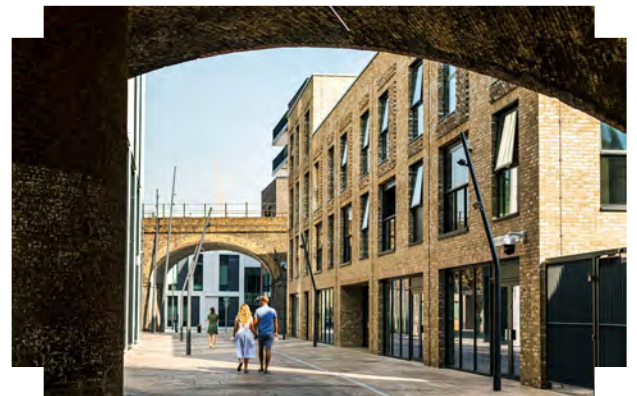
The building subtly steps up in scale to emphasise the corner | Battersea Exchange, London
