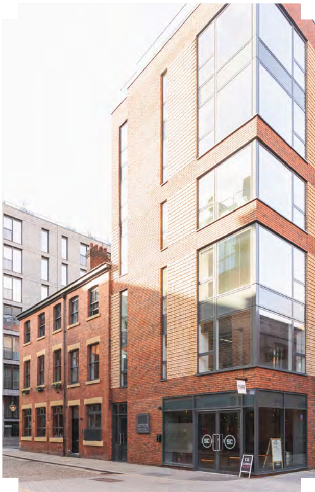
A sensitive, contemporary response to heritage which steps up to the corner | Ancoats, Manchester
