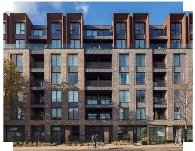
A range of complementary materials, generous windows and inset balconies create depth in the elevation
