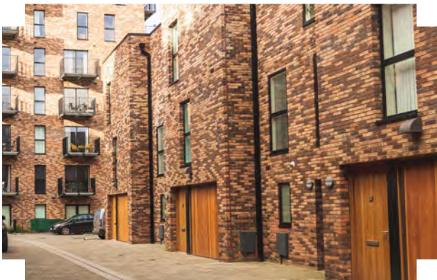
Integral garages within the building footprint, staggered and punctuated by ground floor windows | New Islington Manchester
