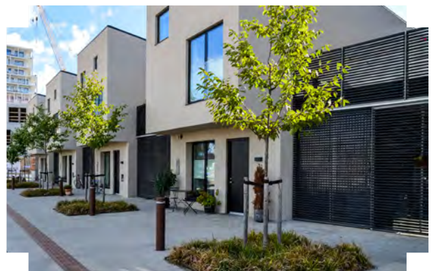
Integral garages punctuated by windows and doors at ground floor, with private roof terraces above | Nordhavnen, Copenhagen
