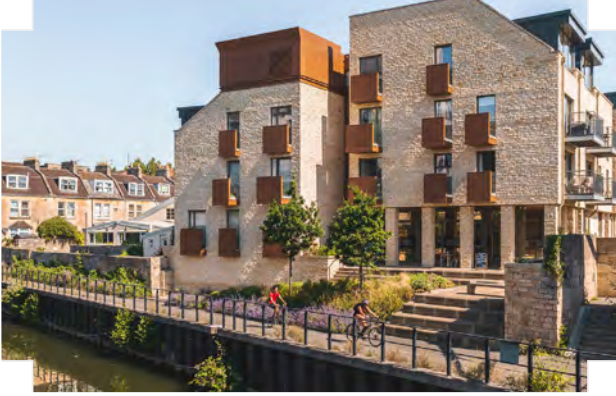
Split-level building steps up with the topography of the slope | Bath Riverside, Bath
