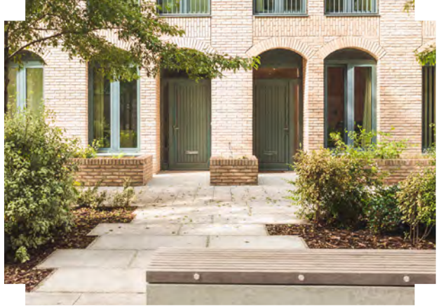
A narrow, low-set building threshold and recessed front door creates defensible space, whilst retaining visual connection between home and street | Embassy Gardens, London
