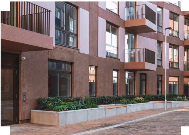
Multifunctional building threshold creates privacy, integrating seating and green infrastructure creatively | Sugar House Island, London
