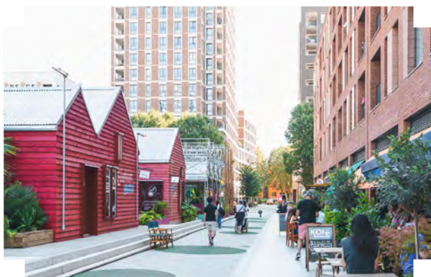
A range of low-rise structures house businesses along a pedestrian-priority street | Elephant Park, London
