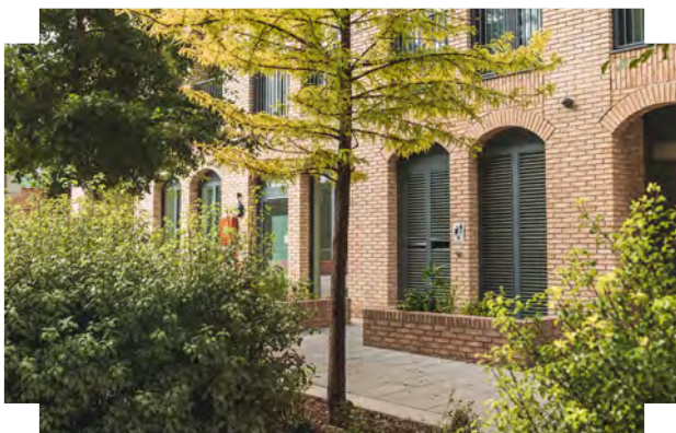
Subtly integrated plant facilities and bin stores at ground floor level | Embassy Gardens, London
