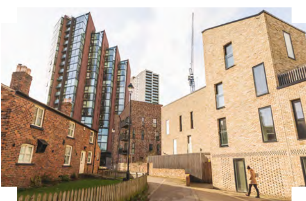
Building entrances and roofscape step with topography, creating visual interest | New Islington, Manchester
