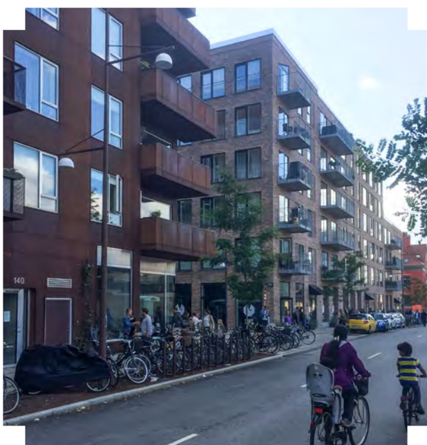
Medium-rise apartment blocks incorporate dual aspect apartments, large balconies and active ground floors
