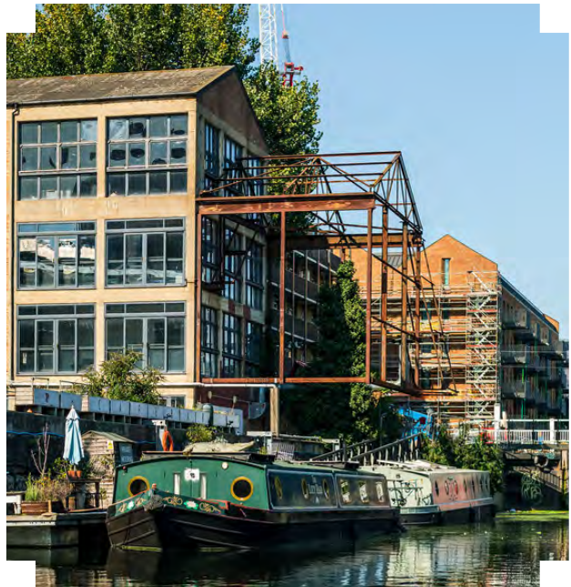
Converted industrial buildings to the rear of the image address the riverfront | London
