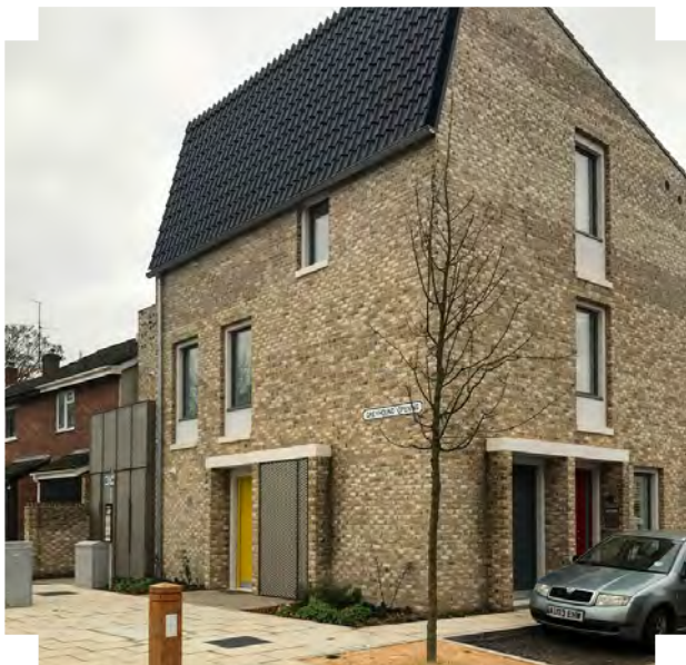
Small-footprint apartment building bookends a row of terraced housing, appearing as a natural extension of the terraced row | Goldsmith Street, Norwich
