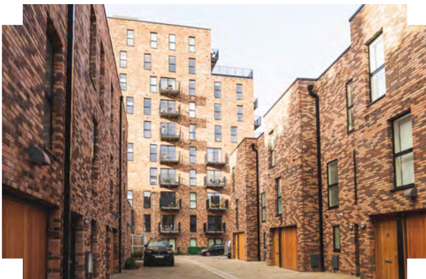
A range of tenures and typologies mixed as part of a tenure-blind neighbourhood block New Islington, Manchester
