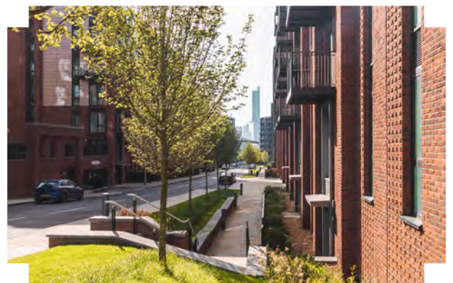
A combination of steps at the top of the slope and a level route at the lower level provides access to the building for people with different levels of mobility | Middlewood Locks, Salford
