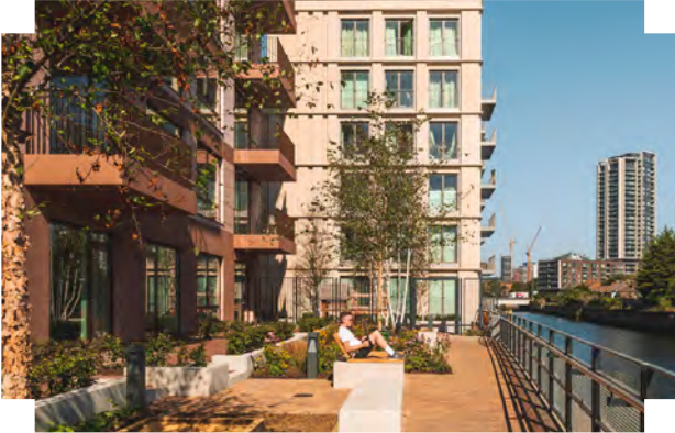
Active frontages, habitable rooms and balconies address the river and adjacent space | Sugar House Island, London
