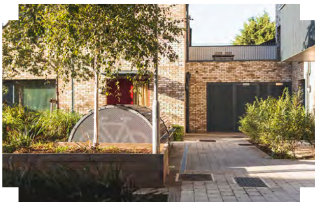
Well-overlooked and secure cycle store, considered and delivered as a fundamental element of the residential courtyard space | Wharf Road, London
