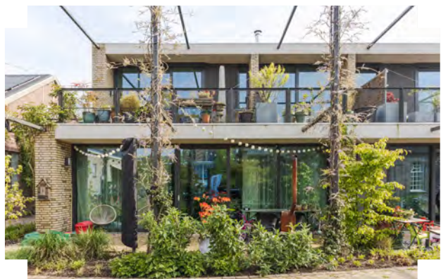
Vertical elements in the landscape and along walls allows plants to climb the building | Eindhoven, Netherlands
