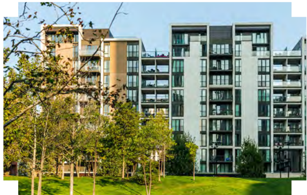
Stepping building line, heights, and recessed balconies create visual interest and depth in the elevation | Victory Park, London
