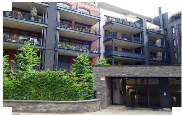
Subtly integrated and well-overlooked underground parking entrance | Dusseldorf, Germany
