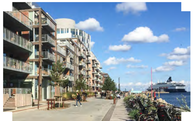
Apartments with large balconies are setback from the water, creating public open space along the waterfront | Nordhavnen, Copenhagen
