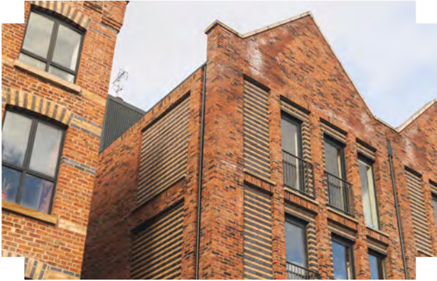
Stepping roof form and gable roof pitches reference historic warehouse buildings and create visual interest Warehaus | Ancoats, Manchester
