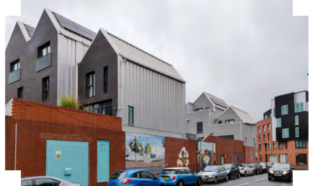
Roof form and materiality complement the areas heritage
