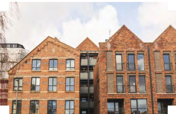
A sensitive, contemporary response to the historic warehouse building | Ancoats, Manchester
