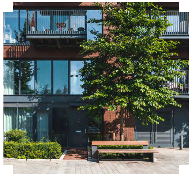
Apartment block integrates townhouses at lower floors, with apartments above. Protruding balconies are delivered three-storeys up, to ensure a positive space below | City Island, London
