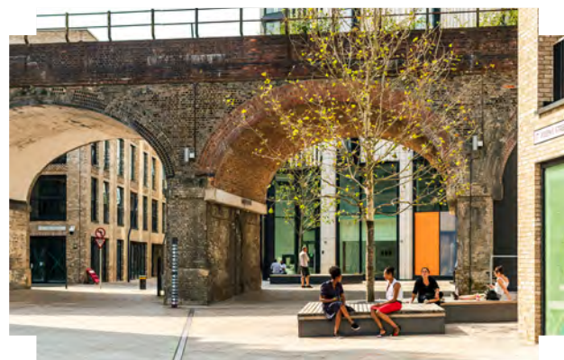
Apartment buildings setback from the viaduct, creating public spaces at the base of the heritage asset | Battersea Exchange, London
