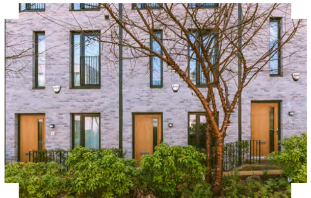
Front doors and large windows should activate the street along Hillgate | Timekeepers Square, Salford
