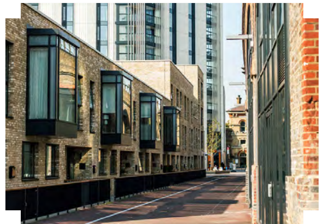
Modern mews dwellings run along a minor street through the centre of the block, contributing to a fine urban grain | Battersea Park, London
