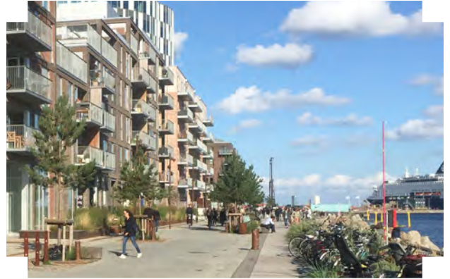
Development is set back from waters edge, creating a pedestrian promenade | Nordhaven, Copenhagen
