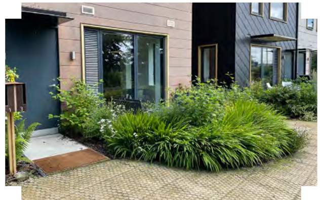
Permeable paving and rain gardens incorporated into the building threshold and streetscene Climate Innovation District, Leeds
