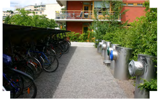
Carefully located pneumatic hatches, subtly integrated into public space and overlooked by surrounding apartments | Hammarby Sjostad, Sweden
