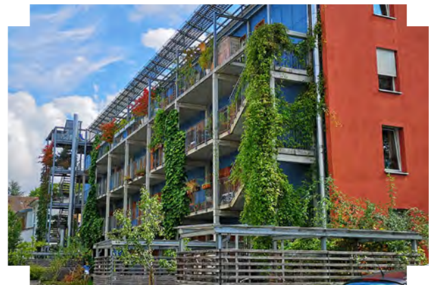
Vertical greening climbs up building and ancillary structures, such as external bin or cycle stores | Vauban, Freiburg
