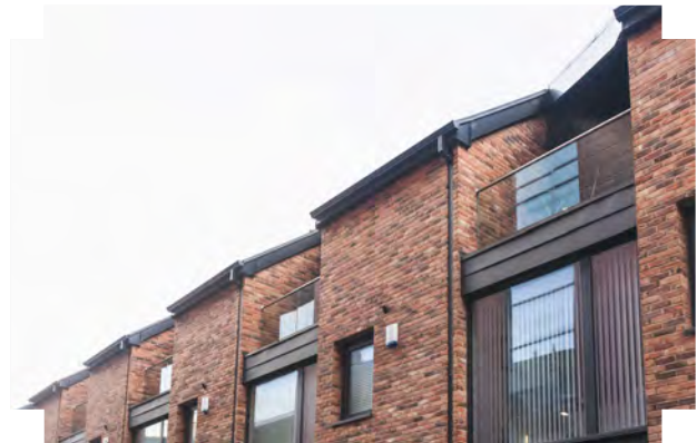
The building line is recessed at roof level to incorporate private amenity space without upsetting the existing building line | Ancoats, Manchester
