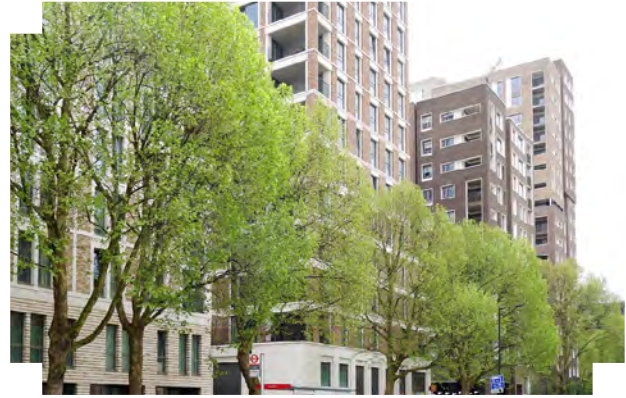
Building heights fluctuate along the perimeter, stepping up to emphasise the corner | King's Crescent, London
