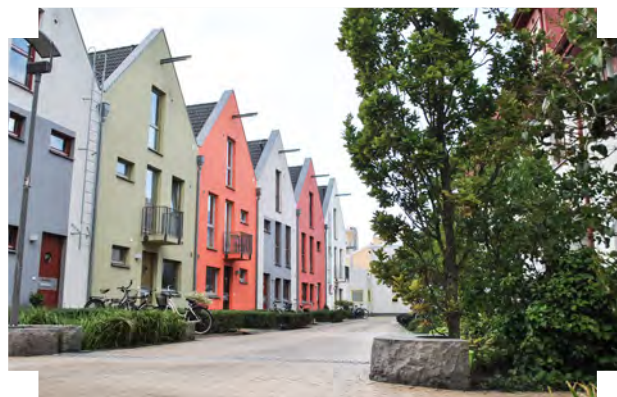
Permeable paving used on tertiary street and rain garden features integrated into design of the street and threshold spaces | Bo01 Waterfront, Malmö
