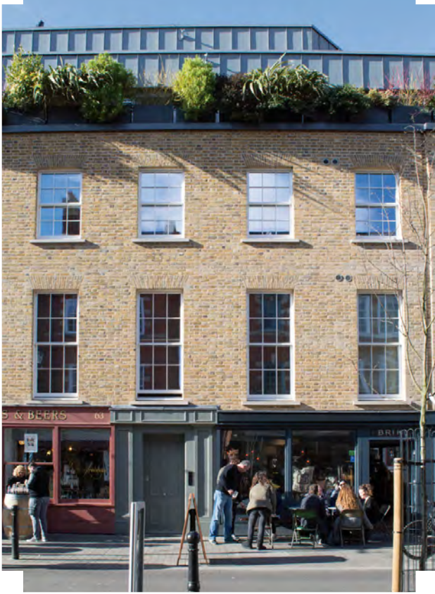
Subtly recessed upper consisting of complementary materials create raised amenity space at roof level | London
