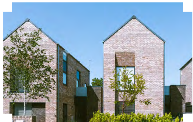
Narrow buildings footprints with staggered upper storey windows limit overlooking between dwellings, and allow a compact urban block | The Gables, Crosby
