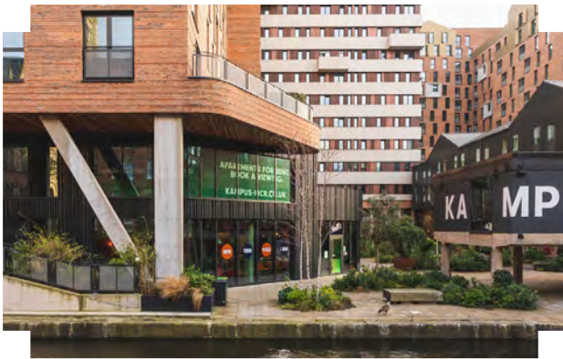
Active uses and recessed upper storeys helps to articulate the lower portion of the building, emphasising a human-scale at street level | Kampus, Manchester
