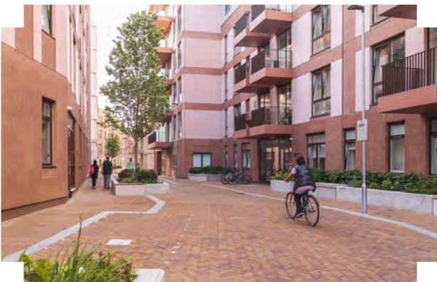
Seating, planting, high-quality surface materials and a flush surface creates a balanced street environment, prioritising pedestrians and cyclists | Sugar House Island, London
