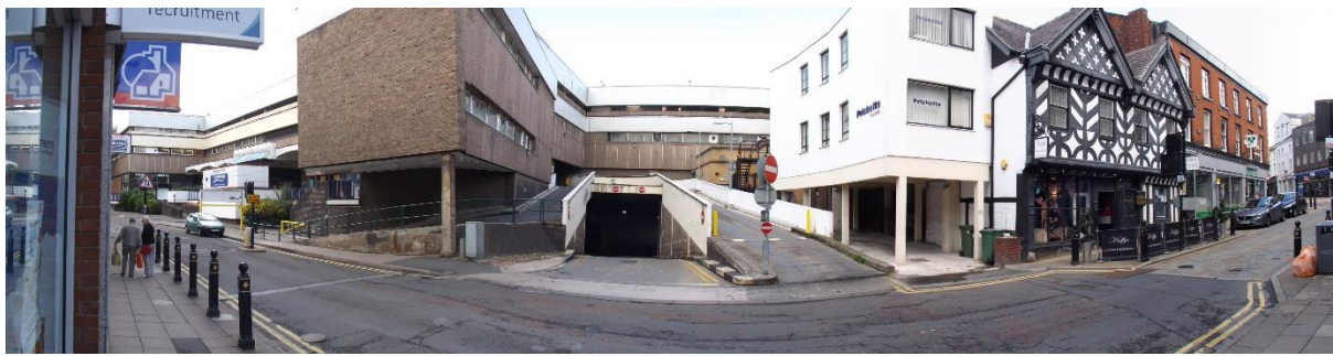
Great Underbank; the complex ramp entry and exit system at ground level for the Merseyway Car Park. Height restrictions have The delivery exit ramp is emphatically signalled as one way because rising plates will damage vehicles mistaking the space as entry only.
